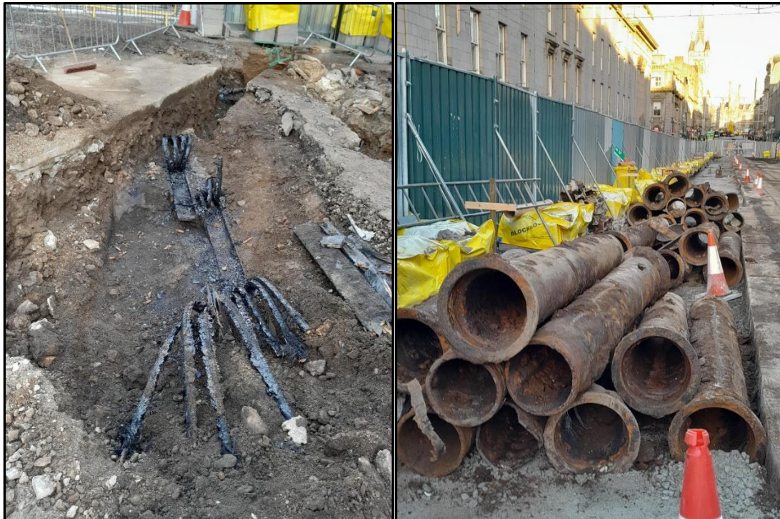
Removal of redundance cables & pipes
