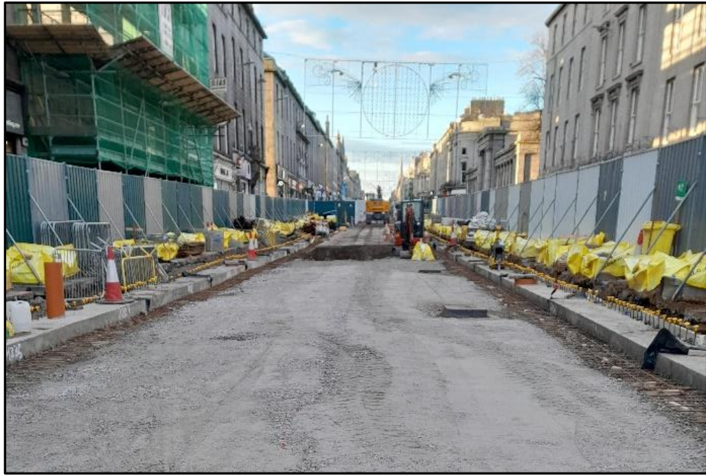
Kerb Log & Preparation of Sub-base
